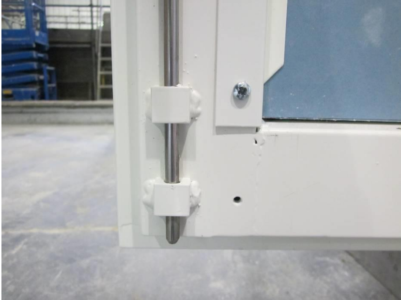
Shoot bolt guide blocks and plasterboard retaining section
