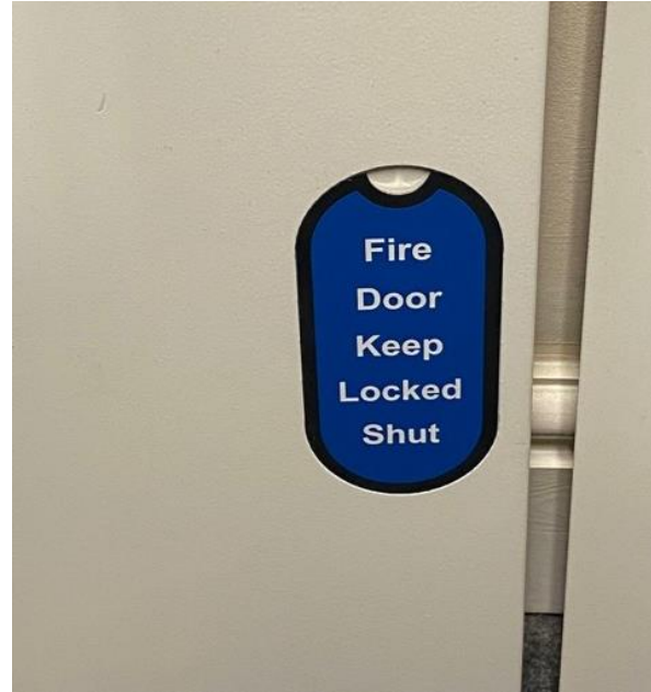
With magnetic fire door sign affixed
